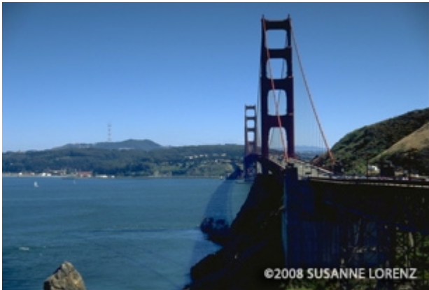
Golden Gate Bridge
